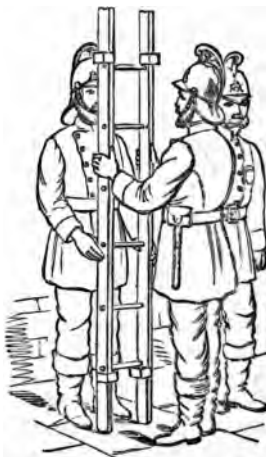
Preparing to raise.
